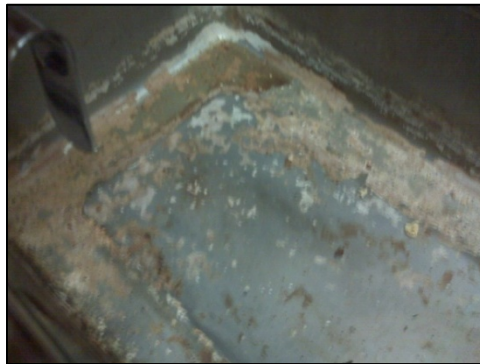
Hard Water Deposits
